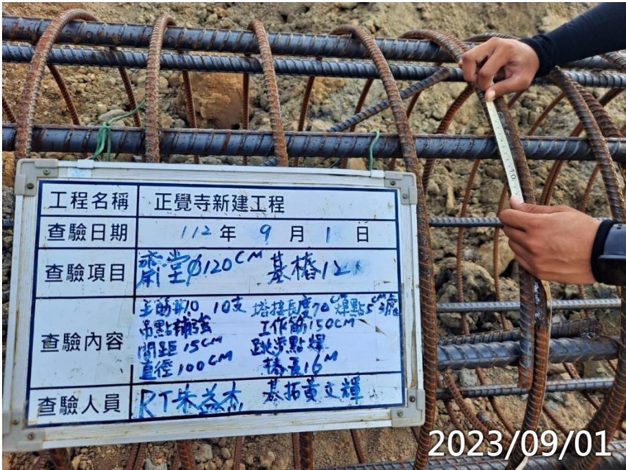
齋堂全套管基樁鋼筋籠查驗
