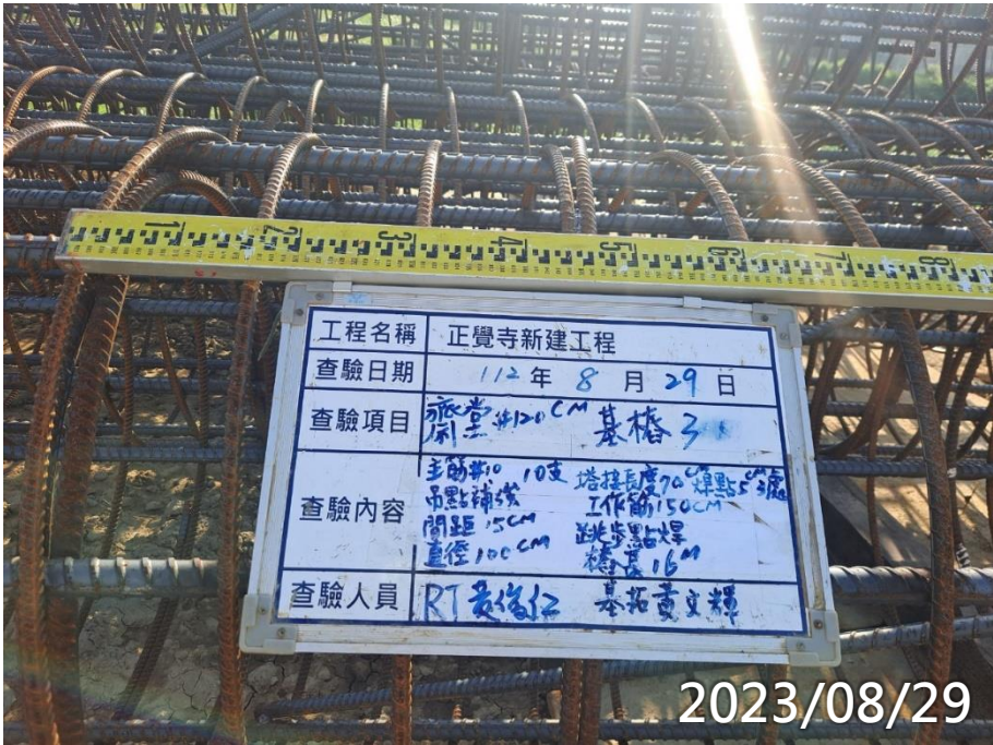
齋堂全套管基樁鋼筋籠查驗
