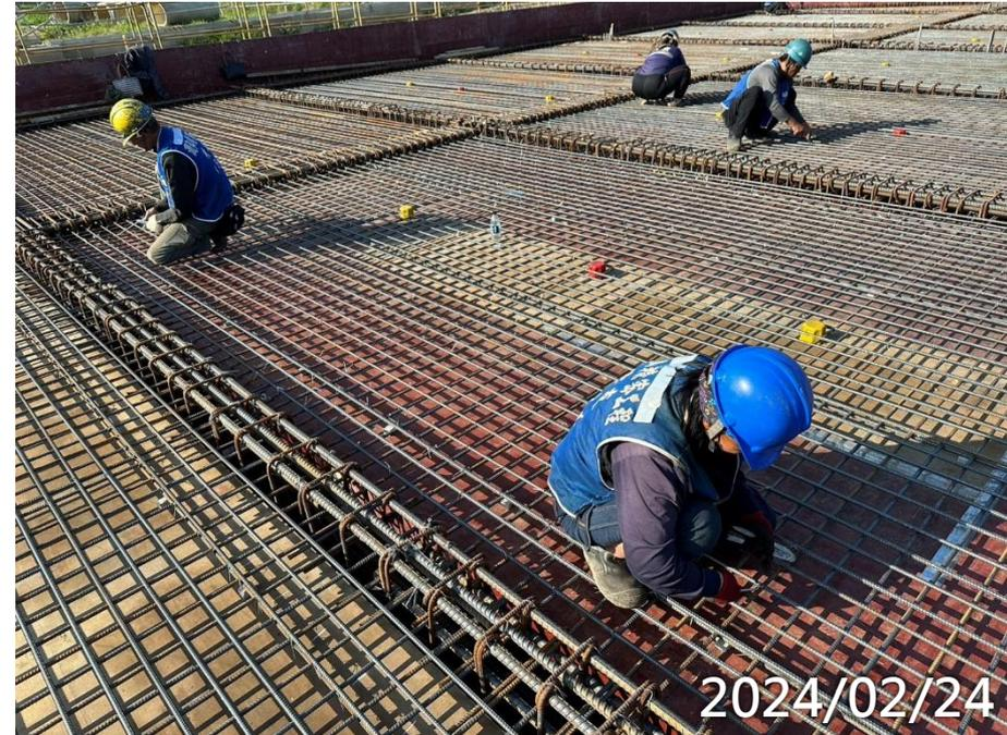
污水廠RF版梁鋼筋綁紮
