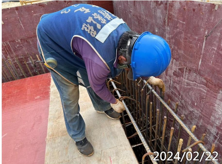
污水廠RF版梁鋼筋綁紮
