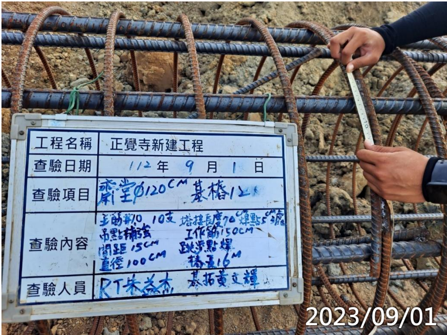
齋堂全套管基樁鋼筋籠查驗
