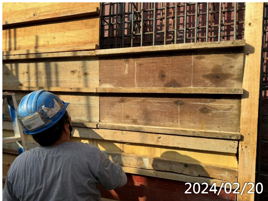
污水廠B1F牆柱模板組立
