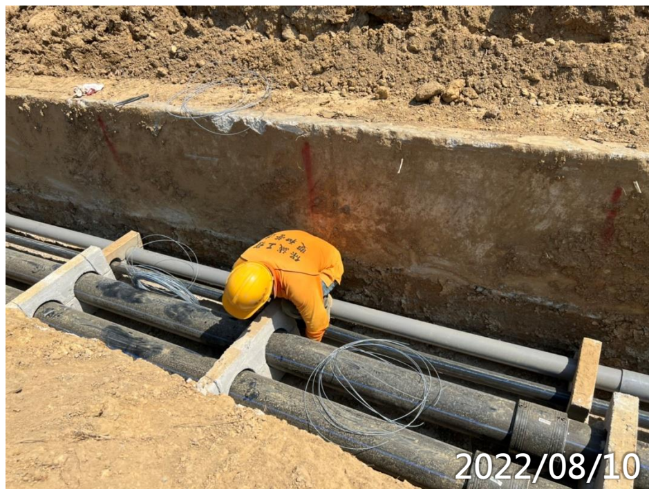
CM5至CM6給水管路配設
